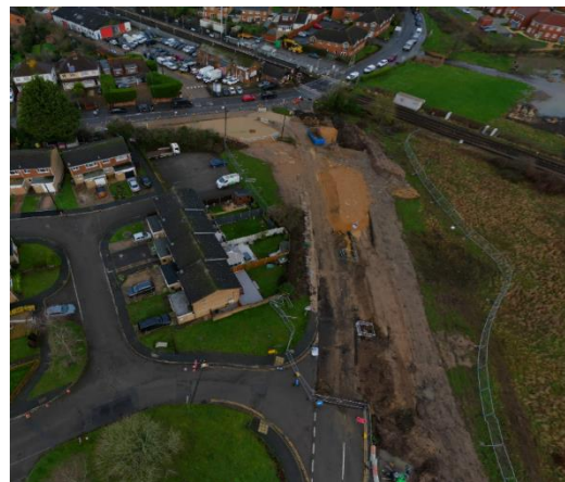
Widening Foreman Road
