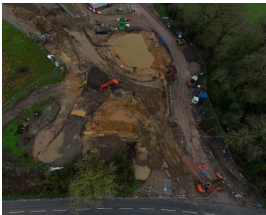
Foreman Road roundabout
