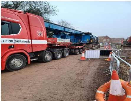
Piling rig arriving on site
