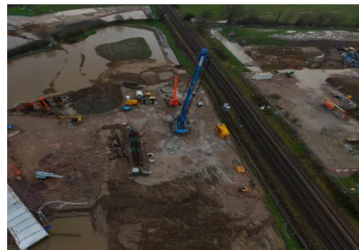
Piling rig in action
