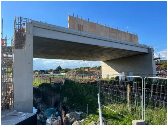
The new bridge
