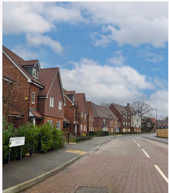
Figure 74: Consistent rooflines, building lines and levels of setback create a coherent streetscene, Hammersley Drive.
