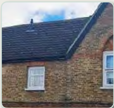
Yellow brick with decorative red brick pattern
