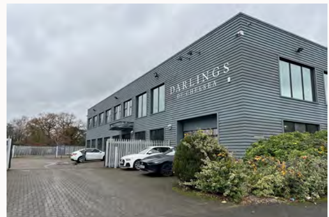
Figure 44: Darlings of Chelsea office unit with a flat roof, grey panelling and large windows to help maximise sunlight, Station Road West.
