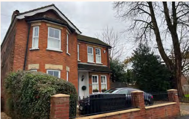
Figure 118: Red brick Victorian detached house with stone lintels above sash windows, Frimley Road.
