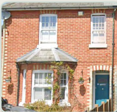
Red brick with decorative quoins
