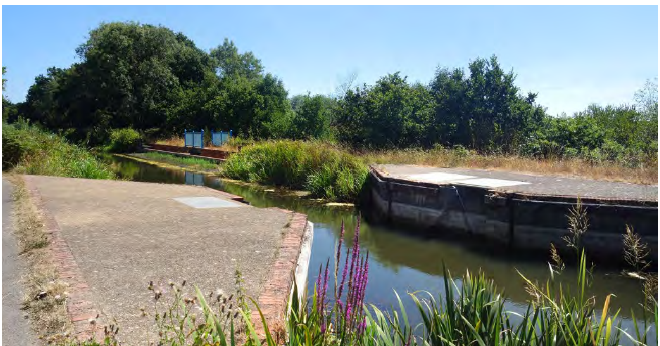
Figure 27: Stop gates by the aqueduct on Basingstoke Canal.
