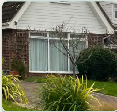
Large floor-ceiling casement window
