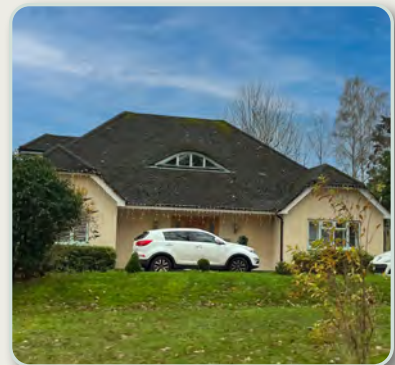
Cross-hipped roof with clay tiles and eyebrow dormer
