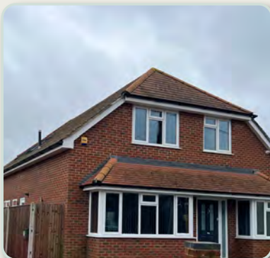
Clay tile clipped hipped roof
