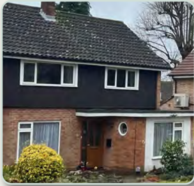
Buff brick with black weatherboard
