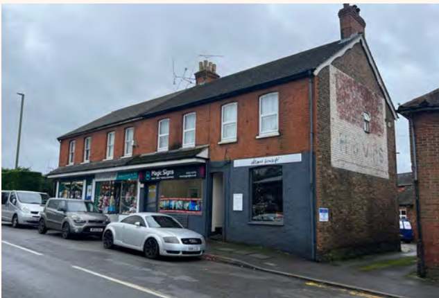
Figure 114: Victorian terraces converted into shops at the ground floor level on Ash Hill Road.
