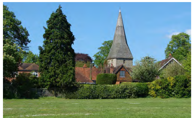
Figure 11: Grade II* listed St Peter's Church, Ash Church Road. (Source: ©Alan Hunt via Geograph)
