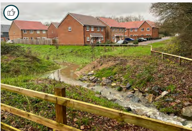
Figure 77: Positive local example of a swale in a recent development to the north of Ash Green Meadow, acting as stormwater runoff attenuation during a rainy day.
