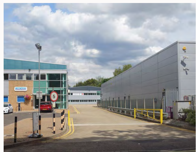
Figure 49: Clearly demarcated entrance with wide roads for the ease of access for HGVs, Lysons Avenue.
