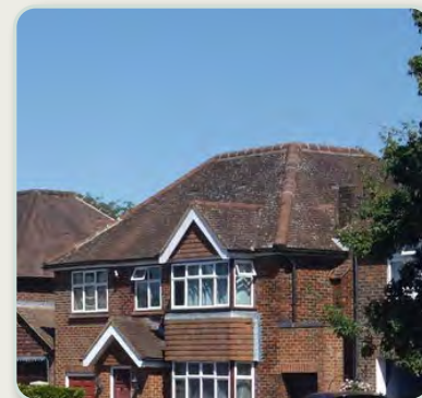
Clay tile hipped roof
