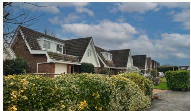
Figure 61: Houses are typically bungalows with steep pitched gable roofs and dormers in Ash Green.
