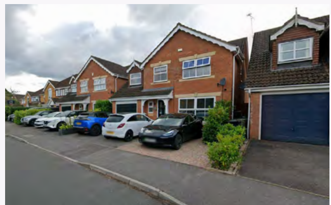
Figure 78: New developments should avoid having over hardscaped front gardens and driveways, which can lead to greater flood risk from surface runoff, Vickers Road.
