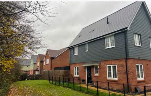
Figure 72: Subtle variation in style and orientation of houses creates a more diverse streetscape.
