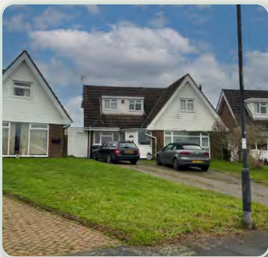
Deep pitched cross- gabled roof with clay tiles
