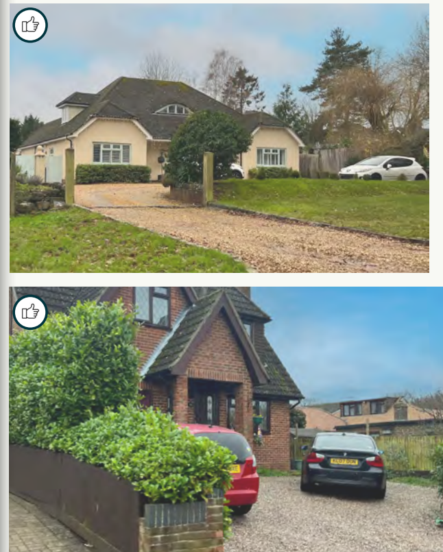
Figure 65: Positive local examples of on-plot parking for properties in Ash Green, for the use of gravel driveways to provide permeable paving.
