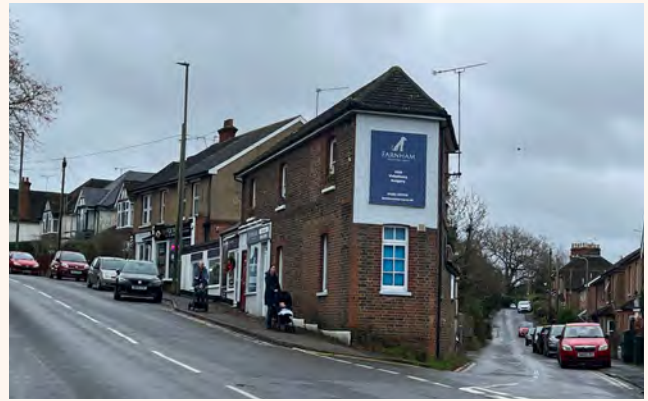
Figure 120: Group of Victorian terraces with ground floor converted as shops on Ash Hill Road.
