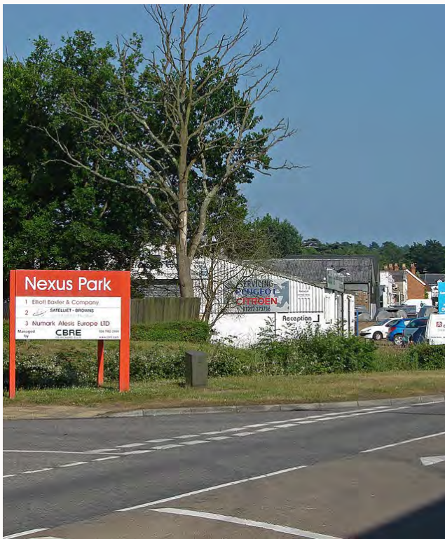
Figure 42: Nexus Park entrance to the industrial area from Lysons Avenue, the positive use of landscaping helps to soften the impact of the large buildings on the streetscape (Source: © Copyright Alan Hunt via Geograph)
