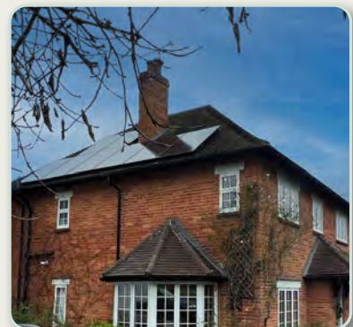
Clay tile hipped roof with solar panels
