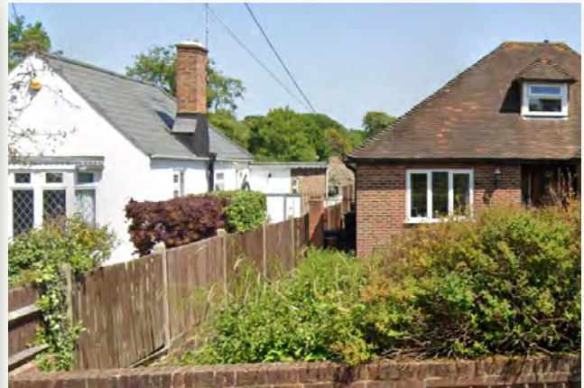
Figure 62: A variety of building materials (brick and render), roof styles (gable and hipped) and vernacular (window types) found within similar neighbouring building types.
